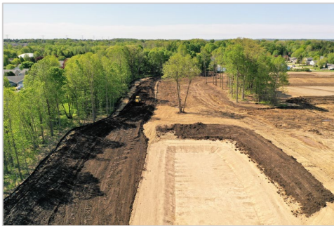
Figure 5 Drone image of Oaks of Jackson construction
