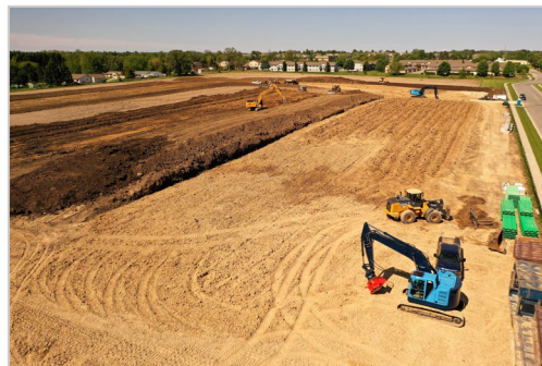
Figure 6 Drone image of Oaks of Jackson construction
